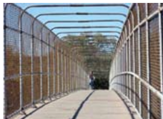
Bicycle and pedestrian bridge with adequate but uninspired design and curvature that limits sight lines; Minneapolis, (U.S.).
