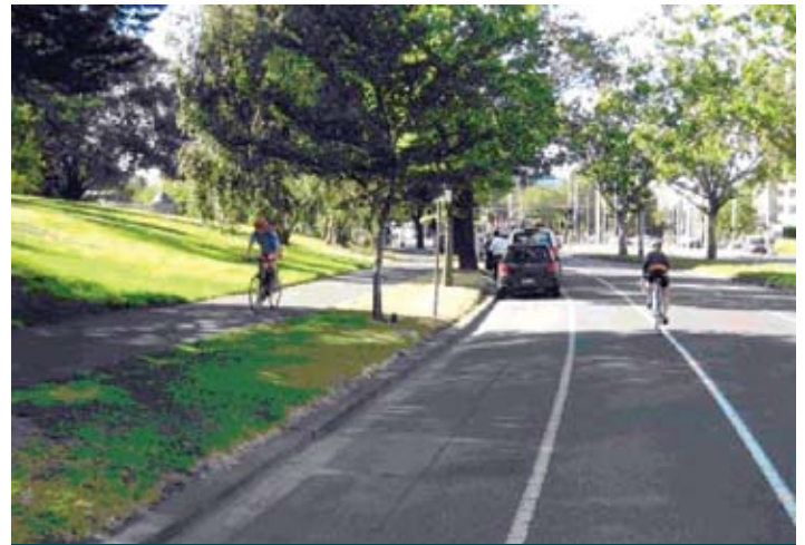
Figure 11: Facilities along St. Kilda Road, Melbourne showing redundancy is fine and sometimes necessary
