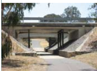
Bicycle (and pedestrian) underpass with clear sight lines; Canberra, Australia.
