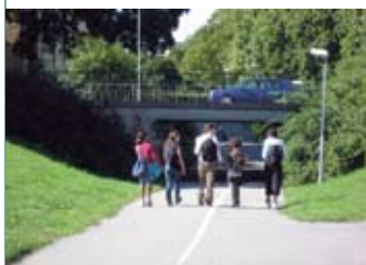
Underpass that is only partially below grade below raised roadway; Vallingby, Sweden. Sight lines are adequate.
